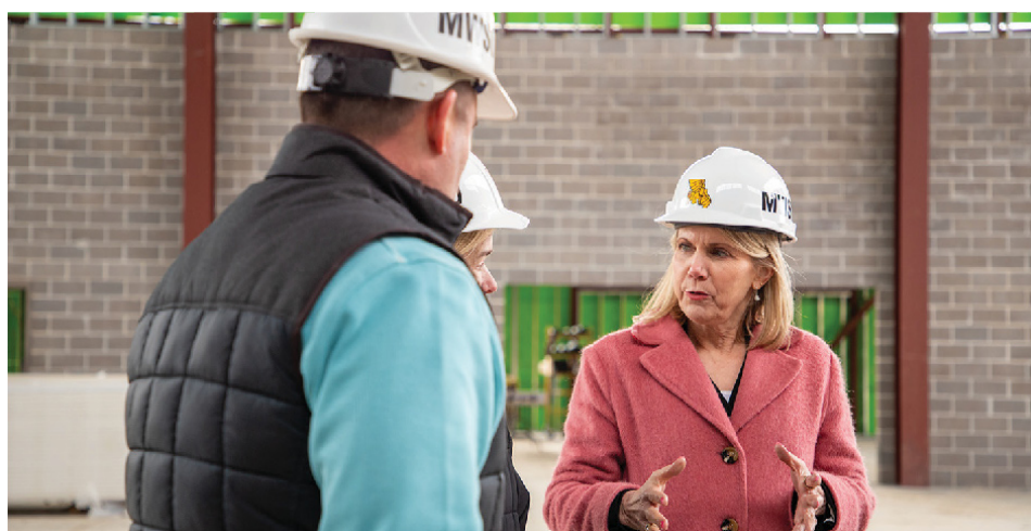
MEETING THE NEED: Elizabeth Kennedy, president of Missouri Western State University, touring the construction site for the new CTAC career training center on campus.
